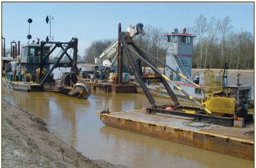
Dredging the Yazoo, Tallahatchie and Coldwater rivers will allow increased flow out of reservoirs, which will decrease the chances of the waterways flooding. This dredging is part of the Upper Yazoo Project.
